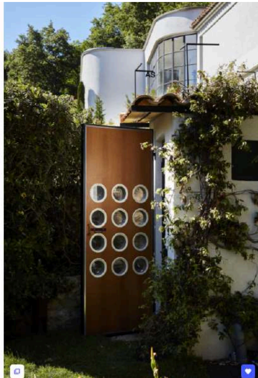
The demountable prefab home, originally designed by Prouvé in 1944, has been adapted into a guest bedroom with a newly attached bathroom created by French architect and designer Charles Zana.
