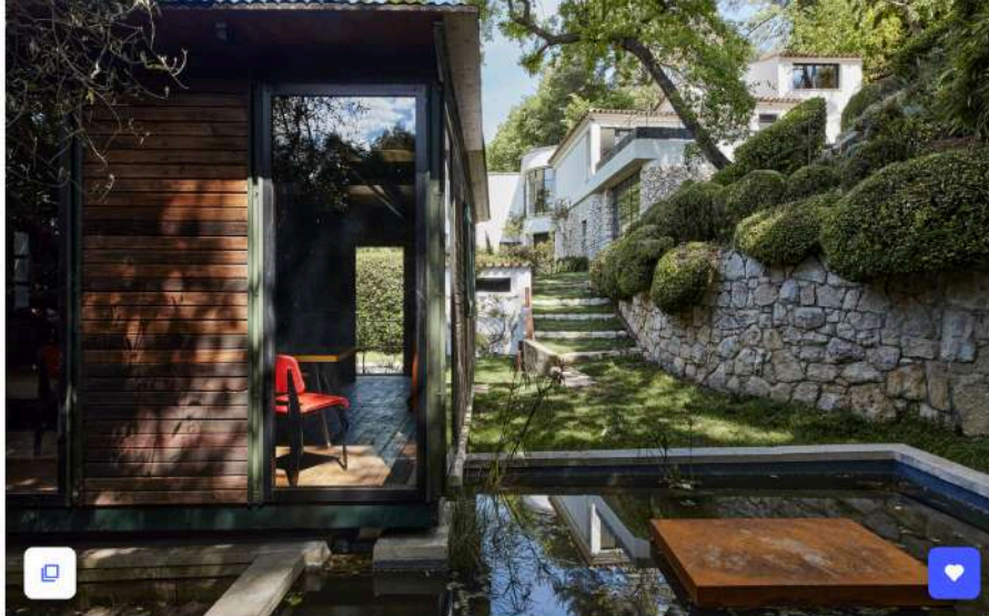
The Jean Prouvé–designed prefab is tucked away in the backyard between two koi ponds.
